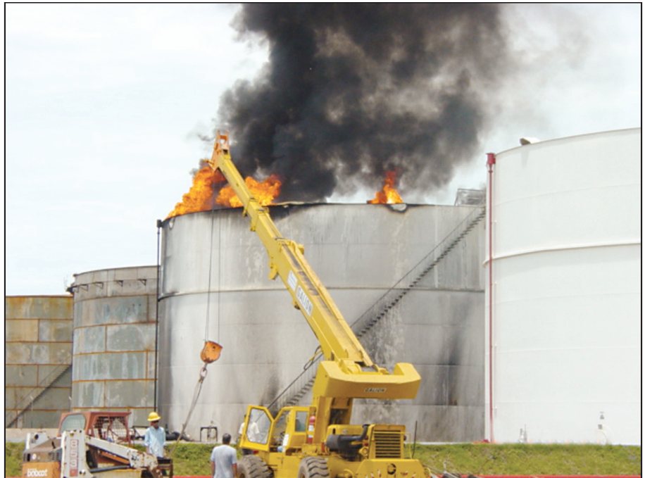
The vapor space within this cone roof tank demands a thorough knowledge of tank construction and fire dynamics — and of course ThunderStorm® ATC!
